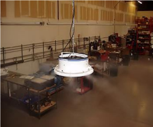
Applications include industrial sites where odor, dust, and humidity control is desired. Misting combined with a proper fan, can provide a high cooling effect.
